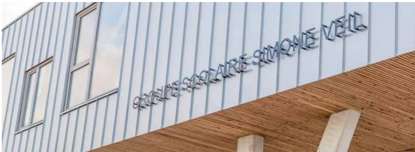
Winkelfalzfassade in Uginox Top. | Foto: © Sandrine Rivie
